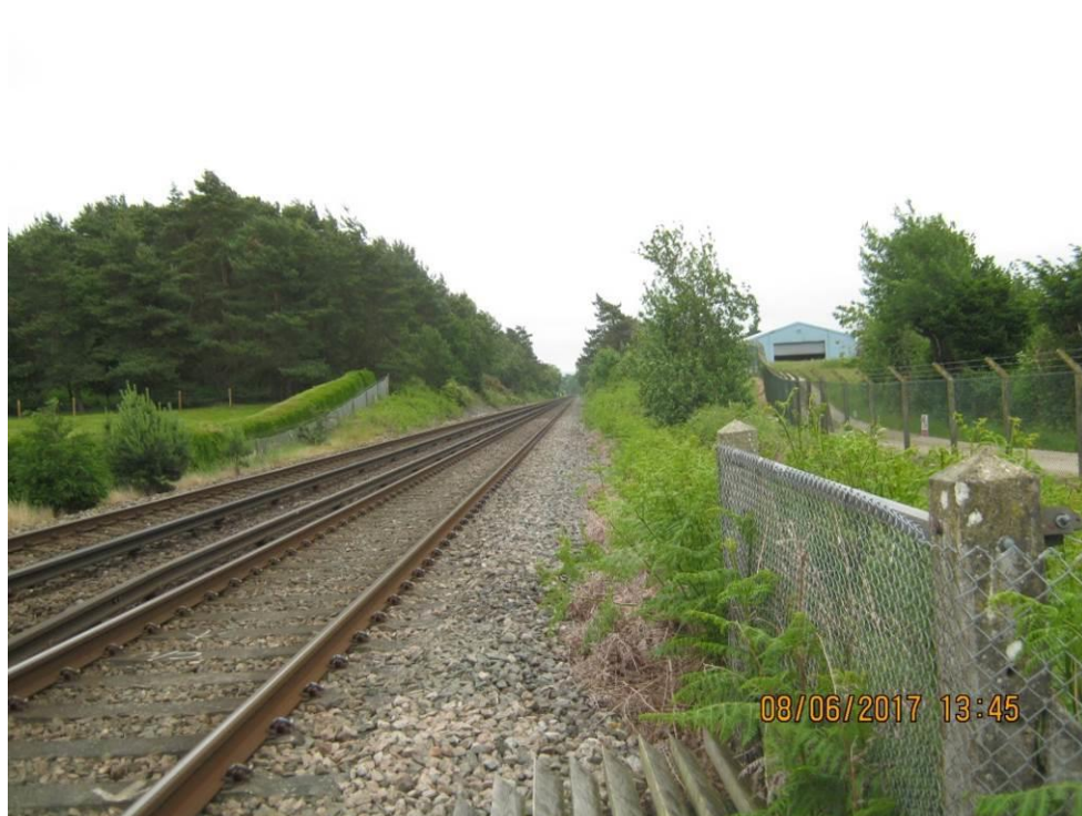
Downside looking towards a down direction train approach
