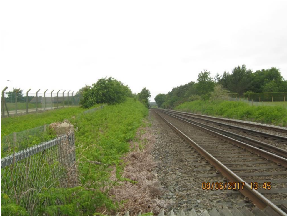
Down side looking towards an up direction train approach
